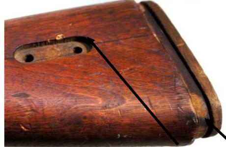
Cut for rear swivel and butt plate but not installed
