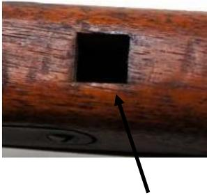
Cut for rod catch but not installed
